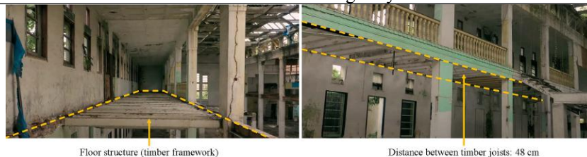
Figure 14. Floor framework on mezzanine level
