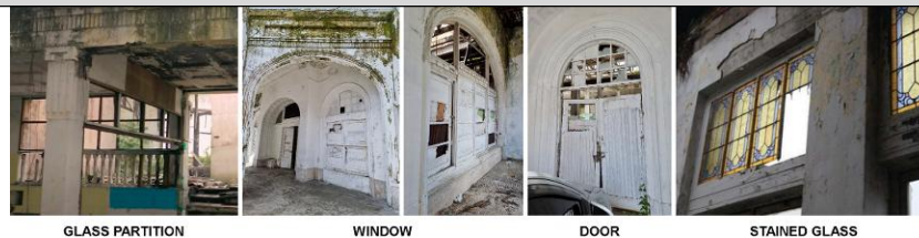
Figure 12. Interior partition and façade of Warehouse
