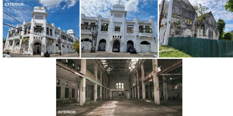
Figure 9. Exterior and interior of Warehouse
