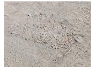
Fig. 5. Intermediate Pothole
