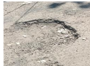
Fig. 6. Severe Pothole
