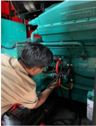
Figure 2 Checking the Generator Set Starter Dynamo
