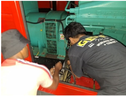
Figure 11 Battery replacement and generator battery charger installation
