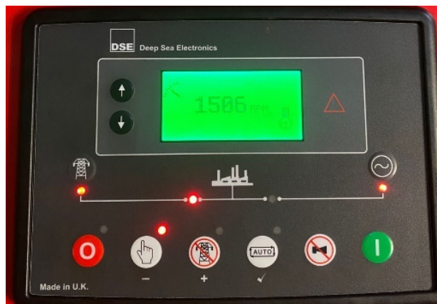
Figure 3 Engine speed (RPM) indicator on the generator control panel during normal operation
